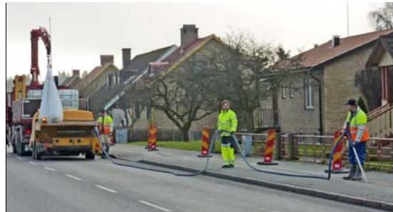
The sawing machine can cross streets without any major obstacles in the traffic. The traffic is released immediately after the sawing machine has crossed the street and the open trench may be crossed by traffic without any problems at all.
