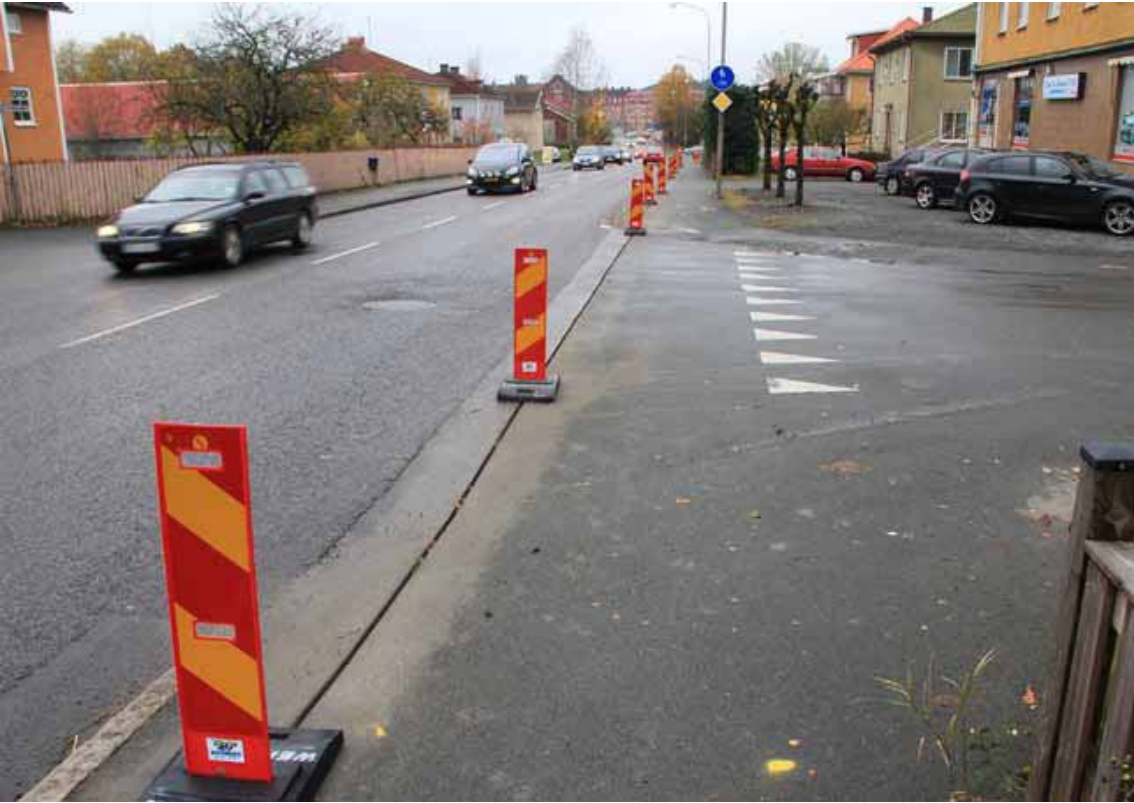
The sawing machine can cross streets without any major obstacles in the traffic. The traffic is released immediately after the sawing machine has crossed the street and the open trench may be crossed by traffic without any problems at all.
